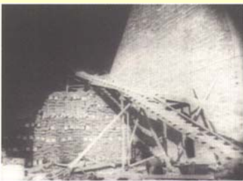
Remove Sandbag, etc. for Barricade at the North Gate
